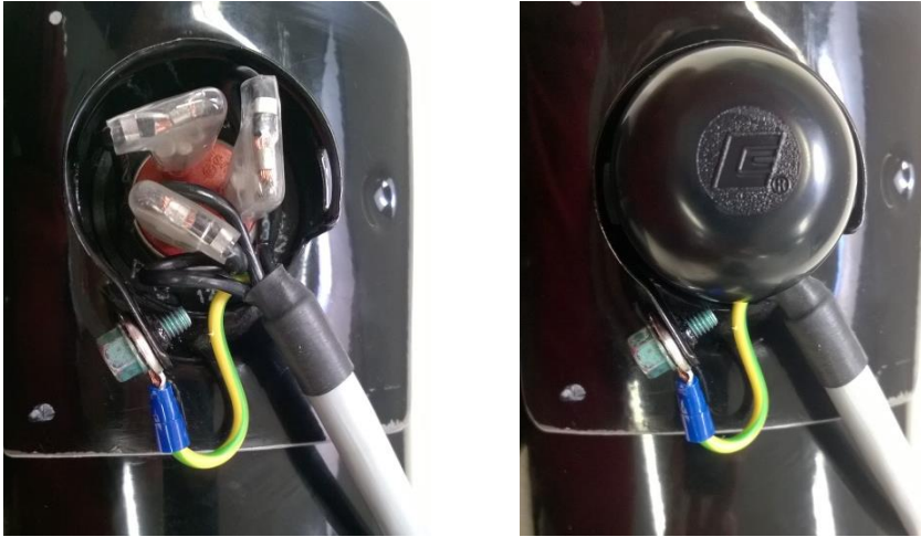
Figure 17: Terminal box and correct electrical installation
