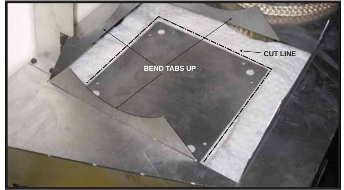
Figure 7.2. Bend Tabs and Cut Insulation.
