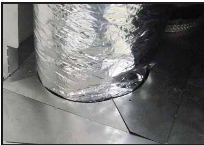
Figure 7.7. Bend Pre-cut Tabs Down.
