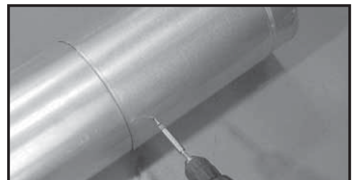
Figure 8.8 Screws into Slip Section
