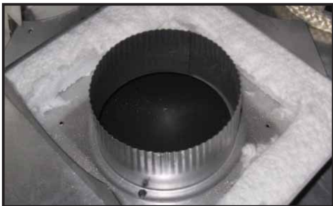
Figure 7.5. Heat-Zone-Gas Collar Installed.
