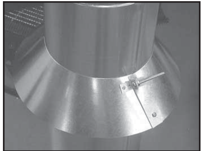
Figure 8.18 Assembling the Storm Collar Around the Pipe
