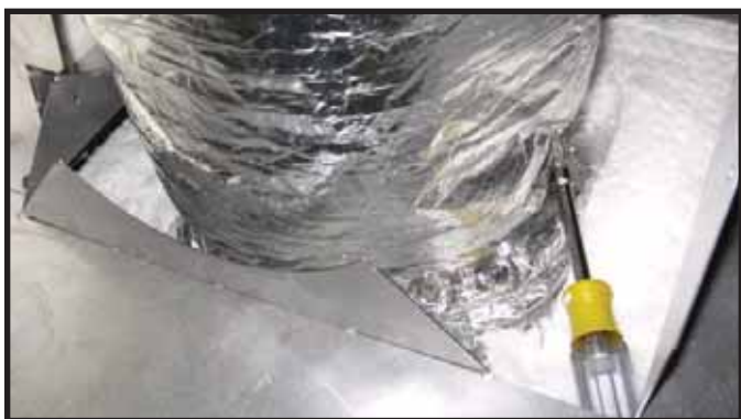
Figure 7.6. Install Insulated Flex.
