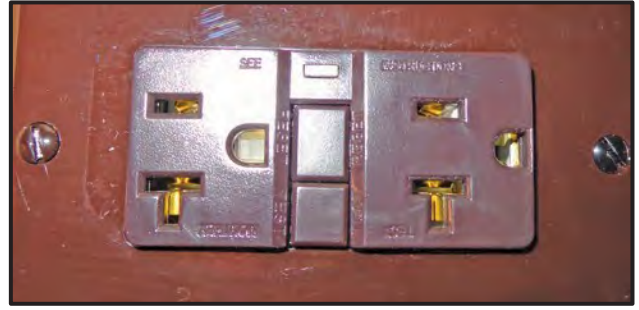
Figure 9-6: GFCI Receptacle
