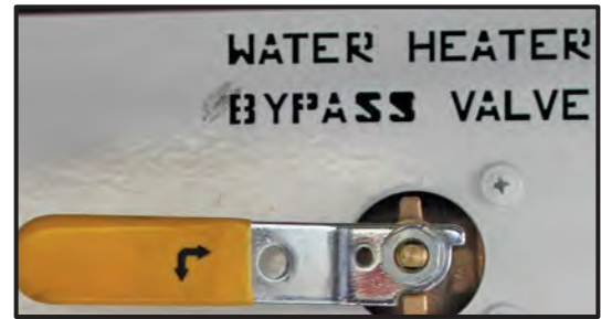
Figure 13-9: Water Heater Bypass System
