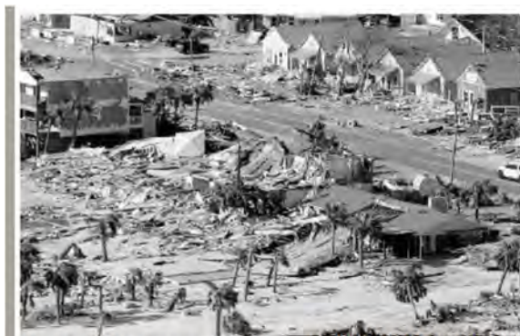
This Oct. 12 photo shows devastation from Hurricane Michael over Mexico Beach, Fla. A massive new federal report warns that extreme weather disasters are worsening in the United States.
