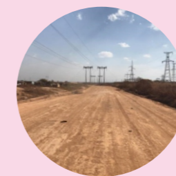
KASAPA road repaired by CDM
