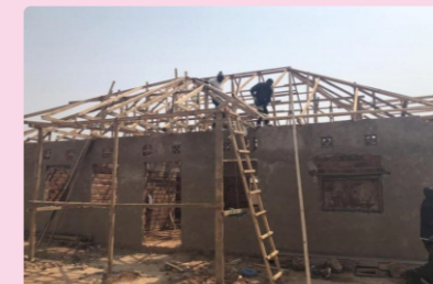
House under construction
