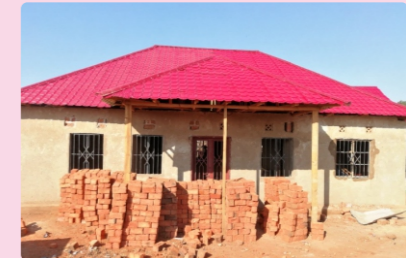
House after renovation
