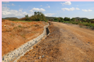
Drainage canal beside road after construction
