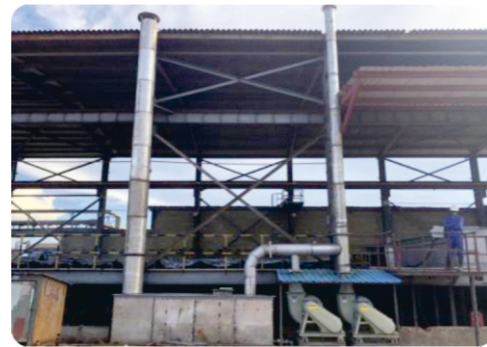
Completed installation of acid mist fan
