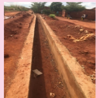
Drainage ditch in KAMATETE
