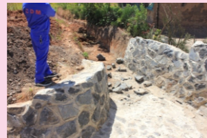
A section of drainage canal in KAWAMA Village
