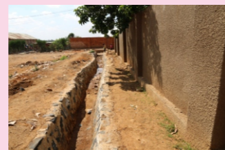
Drainage ditch in the Village
