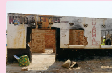
Pharmacy before renovation
