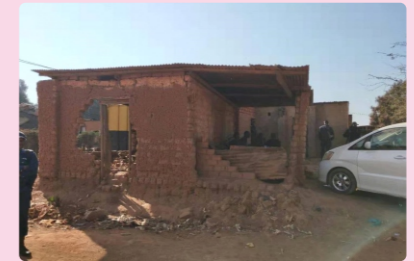
Police station before renovation
