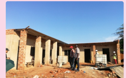
Police station after renovation
