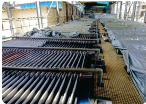
Completed installation of acid gas recovery pipeline
