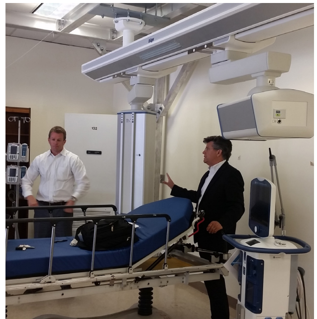
Figure 7 – Ponta Beam installed in mockup at Grady
