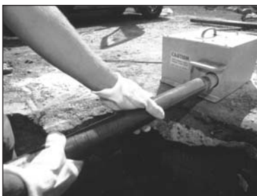
Fig. 5-4. Pipe is typically tapered using one of several power tapering tools available from outside sources.
