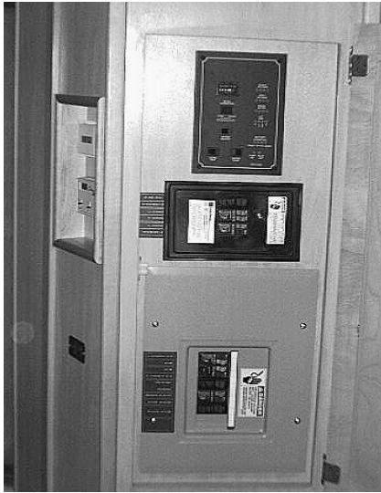
Model 38K or 40J: The 110-volt circuit breaker panel is located behind a cabinet door on the wall in the bedroom.
