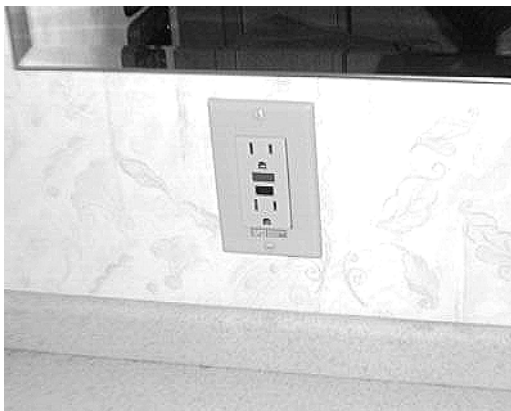
Ground Fault Circuit Interrupter (GFCI)
