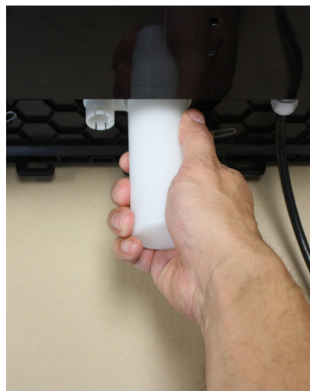
Figure 17: Condensate trap installation
