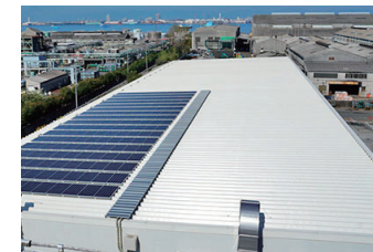
Rainwater collection system on warehouse roof
