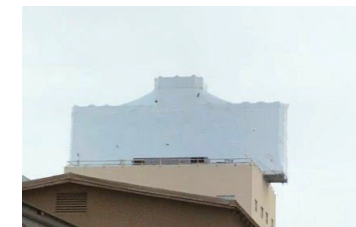
During the roof fall protection
