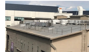
After fall protection
