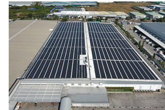
The Chonburi Factory of Sony Technology (Thailand) Co., Ltd. (STT-C)
