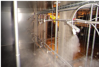
The two-fluid humidification system releases mist
