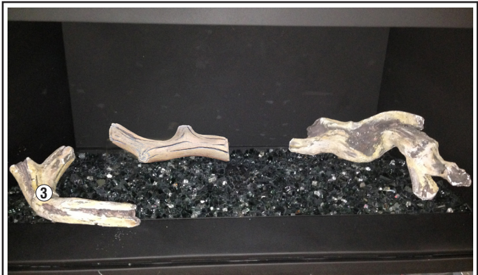
Figure 4 - Place Left Front Log (3)
