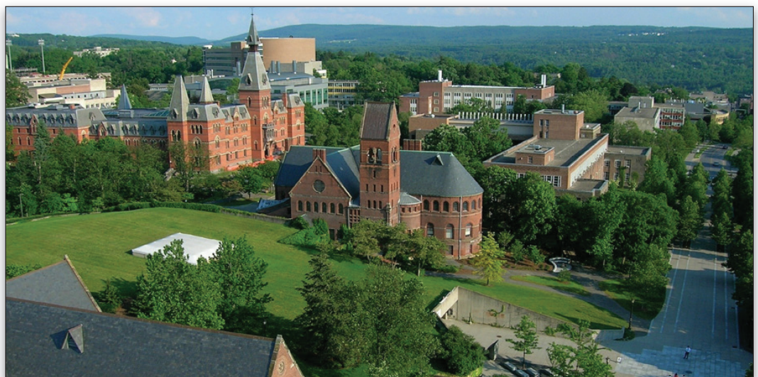
View of the Cornell campus from McGraw Tower with Barnes Hall in the center and Sage Hall to the left.
