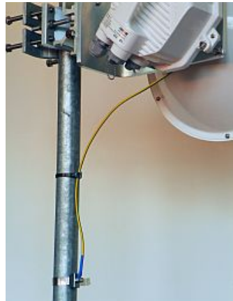
Fig. 4.10: Grounding the RAY unit
