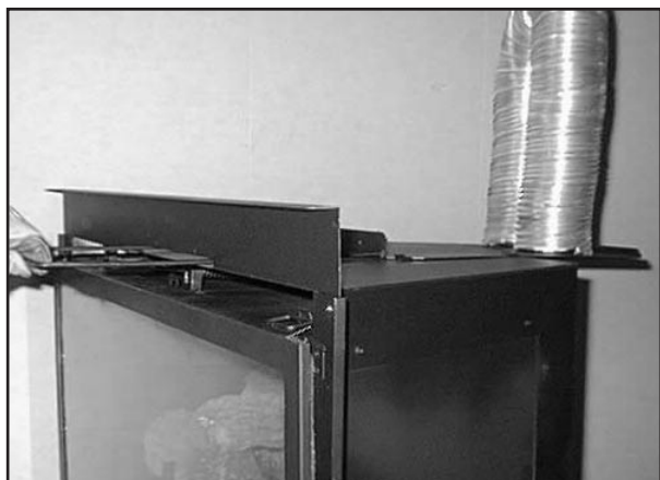
Figure 4 - Reinstalling the Starter Collar
