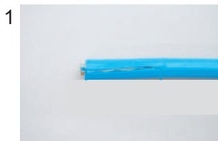
1 Expose inner vinyl sheath.
