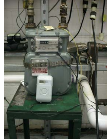
Figure 10 AC-250 gas meter with pulser and readout
