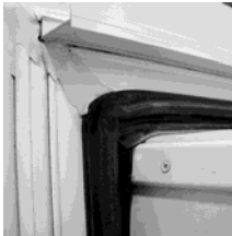
Fig. 5.4 Exterior slideout room corner
