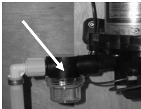
Fig. 8.2 Water pump strainer
