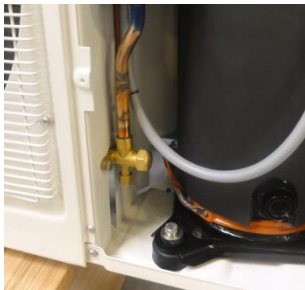
Figure 23: Liquid line service port
