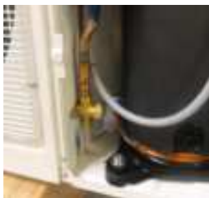
Figure 23: Liquid line service port
