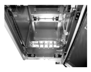
Grid cable entry plate (blank plate)
