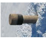
Lighting bollard at Pioneer Park
