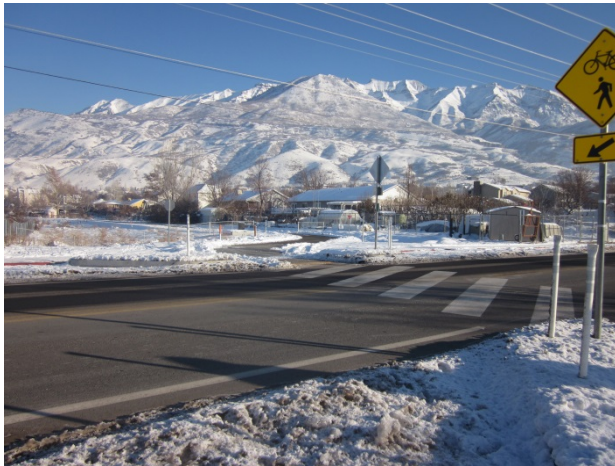
Murdock Canal Trail Crossing and Wayfinding
