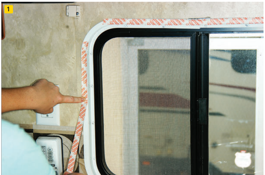
(1) Double-sided tape is applied to the window frame after cleaning. The tape has a strong adhesion but will need to set for 15 minutes before applying the window film.
