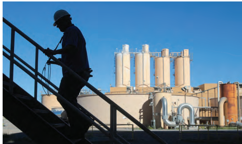
Figure 2: TEP employee Gary Gardner, who is part of the predictive maintenance group, walks throughout the generating station in Springerville, collecting data where he measures ultrasonic, vibration analysis, infrared thermography and electrical motor testing, analyzing equipment to predict when it will need replacing.
