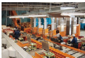
Used air conditioners disassembled at the facilities of Panasonic Eco Technology Center
