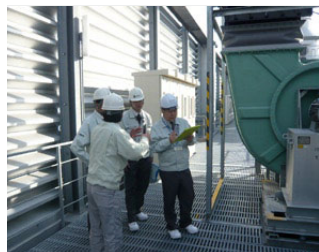
Energy conservation diagnosis
