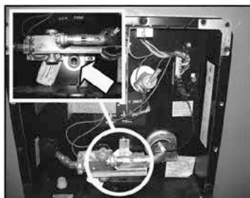
Water Heater Drain Plug Location
