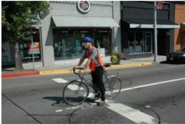
Figure 10: Example of pavement marking at traffic signal that shows bicyclists where to stop to activate the signal. (Source: pedbikeimages.org / Marie Stake).
