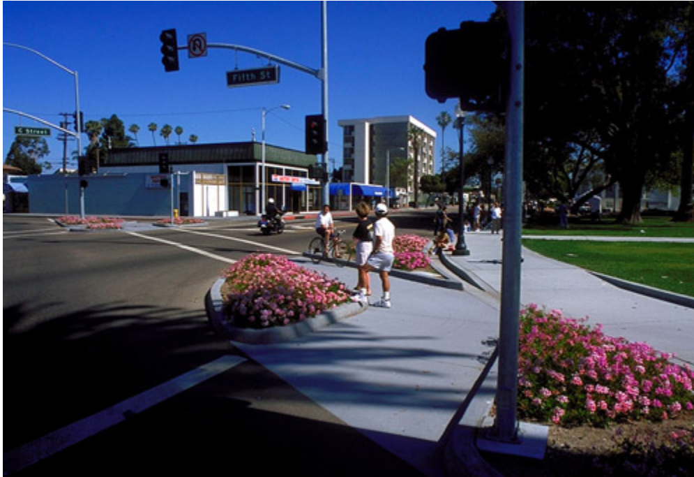
Figure 17. Reduced corner radius at an intersection. Note the location of the previous curb which allowed for higher speed turns by vehicles and increased the crossing distance of the street for pedestrians.
