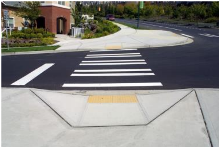
Figure 28. Sidewalk with curb ramps. (Source: pedbikeimages.org / Dan Burden).
