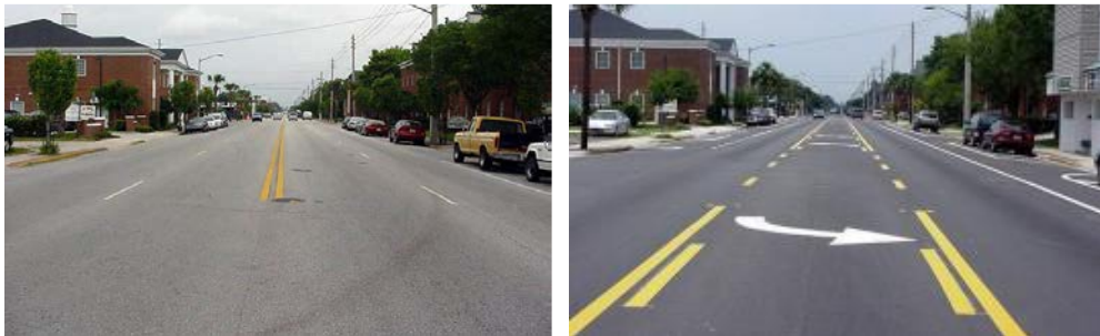
Figure 24. “Before” and "After" picture from a typical four-lane to three-lane conversion. (Source: Federal Highway Administration).
