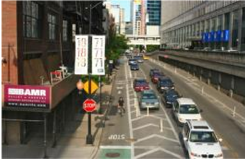
Figure 26. Parked cars and flexible delineator posts on both sides of the street separate the bike lanes from traffic. (Source: City of Chicago).
