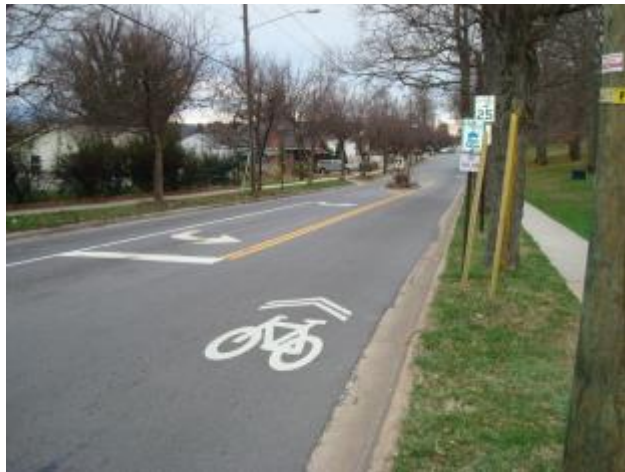
Figure 13. Shared lane marking on a residential street in Asheville, North Carolina. (Source: pedbikeimages.org / Lyubov Zuyeva).
