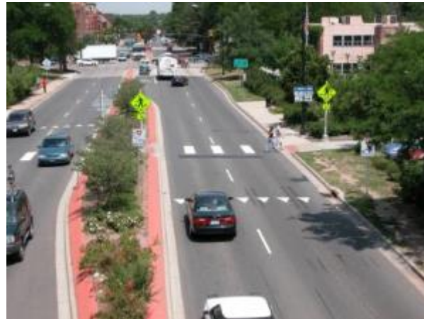
Figure 8. The white triangle pavement markings shown here represent the advance yield line. Some states use a solid white line, as shown in Figure 9. (Source: Toole Design Group).
