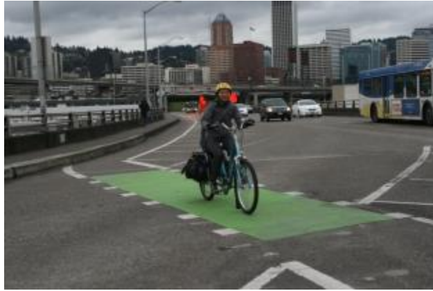
Figure 12. Dashed lines and green paint are used at this complex intersection in Portland, Oregon. (Source: pedbikeimages.org / Shawn Turner).
