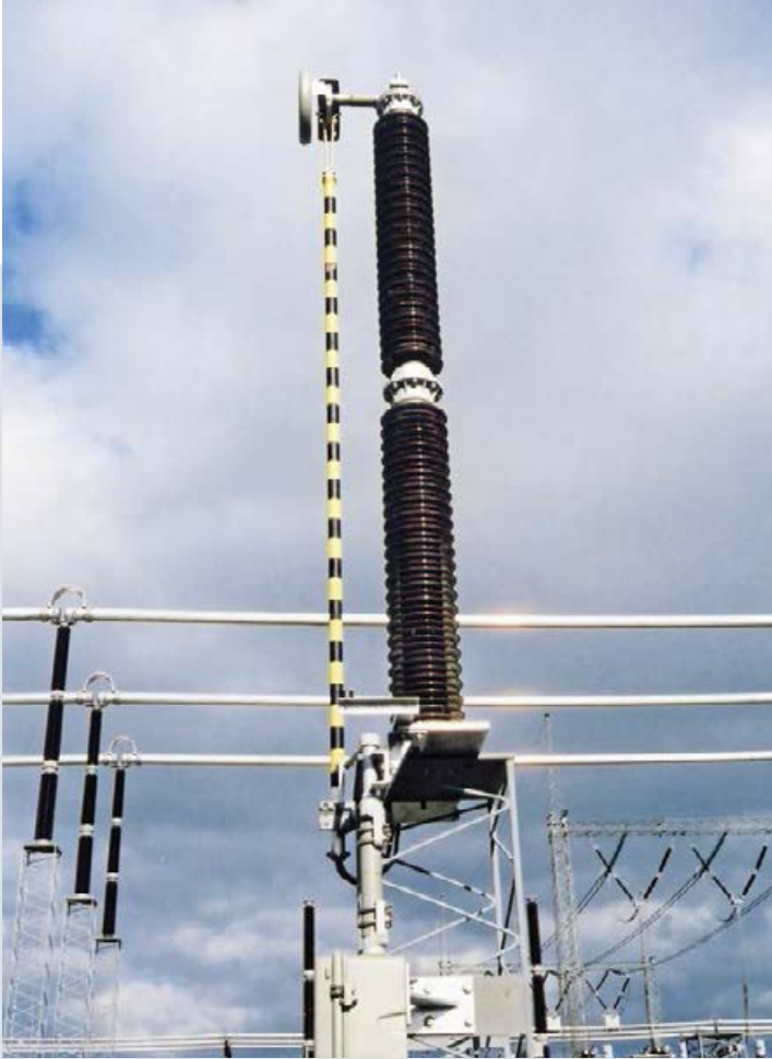
Fig. 30: Free-standing earthing switch
