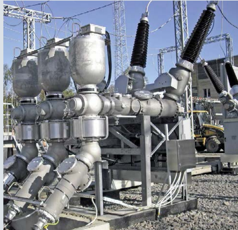
Fig. 20: 3AP1 DTC 145 kV with voltage transformer and cable connection
