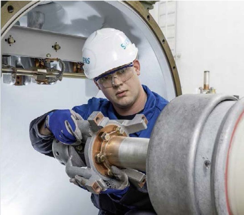
Fig. 106: Contact check of the interrupter unit
