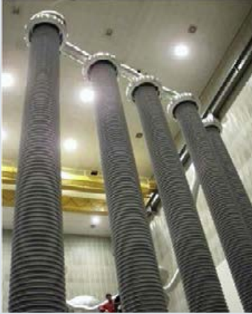
Fig. 54: Energy storage capacitor
