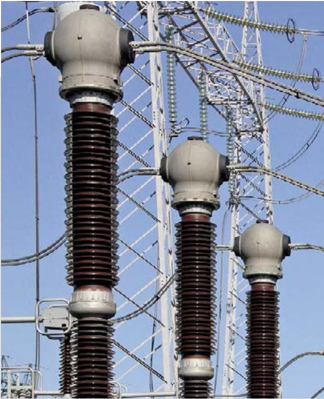
Fig. 44: 420 kV gas-insulated current transformers
