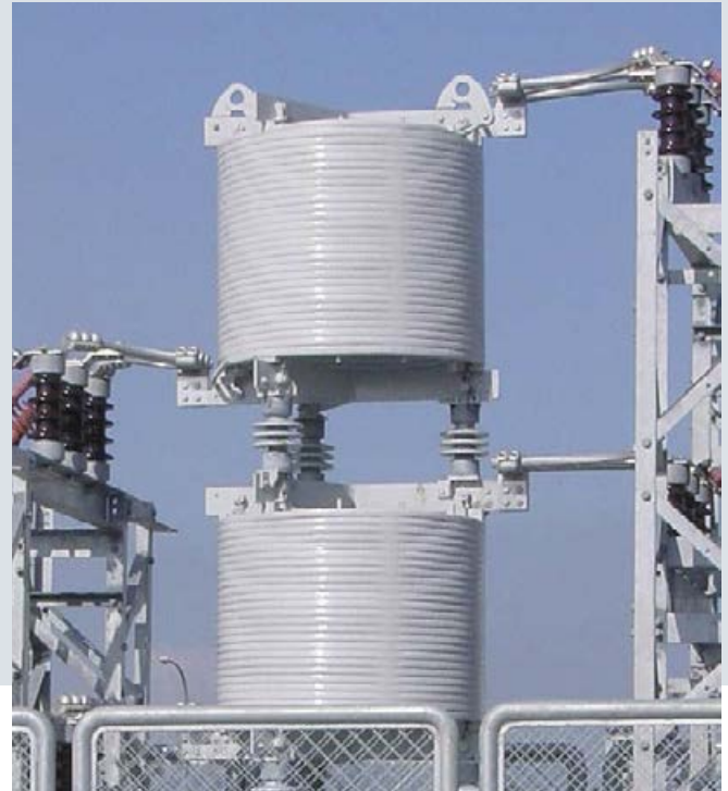
Fig. 66: 3-phase stacked current-limiting reactor
