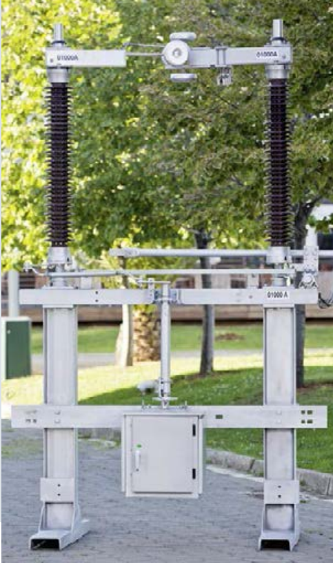
Fig. 24: Center-break disconnector
