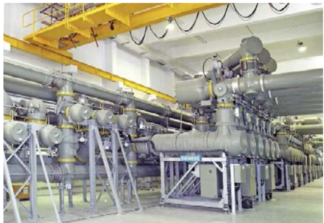
Fig. 91: 8DQ1 switchgear for a rated voltage of 550 kV
