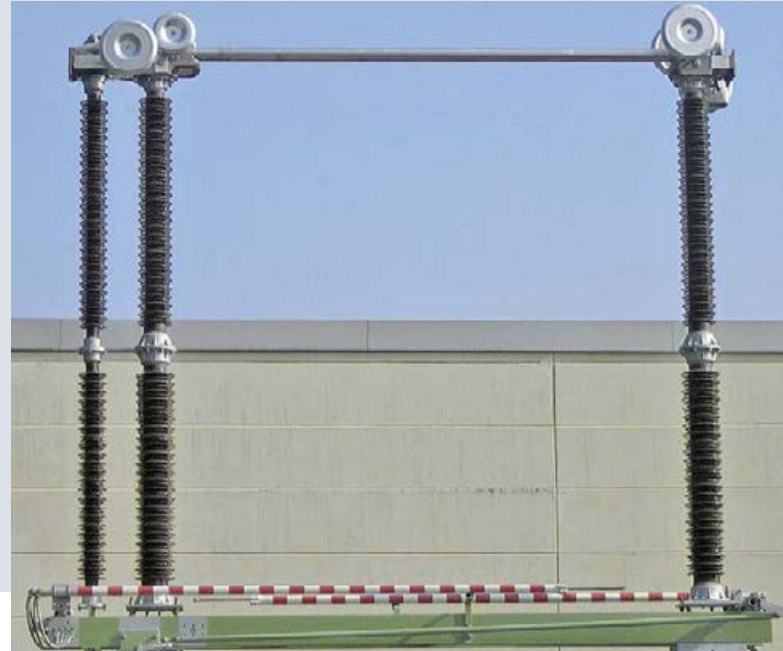
Fig. 27: Vertical-break disconnector
