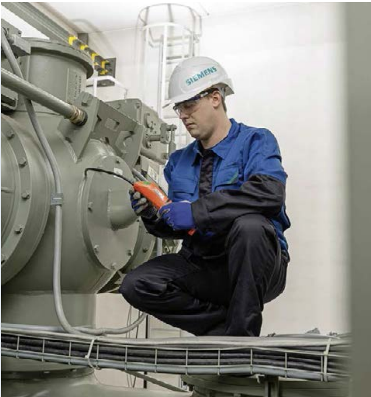
Fig. 105: SF 6 tightness test
