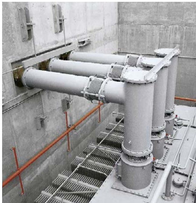
Fig. 98: Transformer termination
