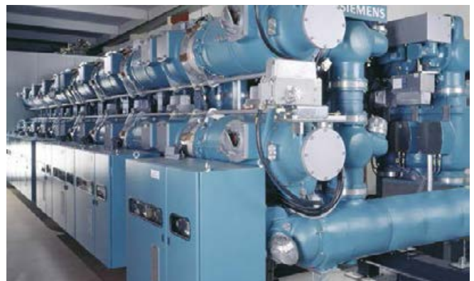
Fig. 89: 8DN9 switchgear for a rated voltage of 245 kV, with a 3-phase-enclosed passive busbar
