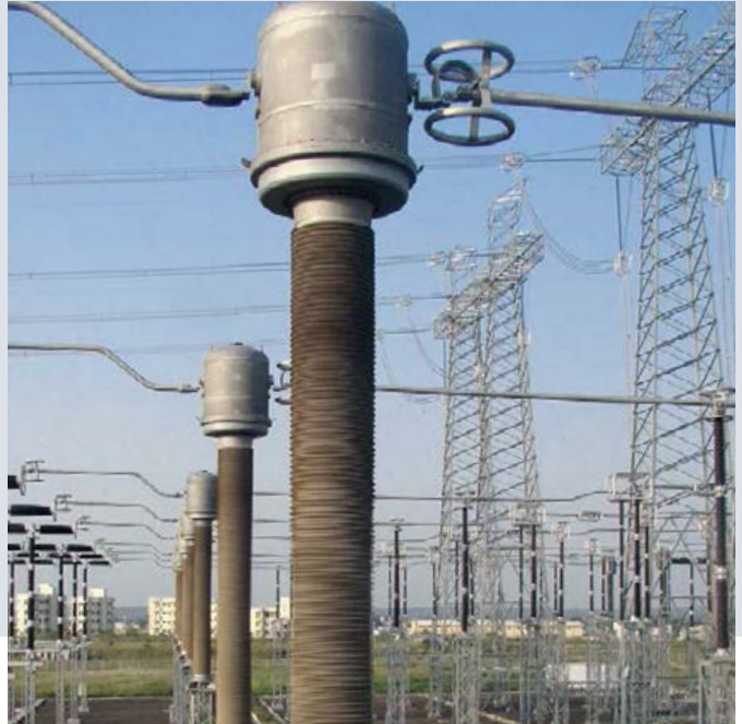
Fig. 45: 800 kV gas-insulated current transformers
