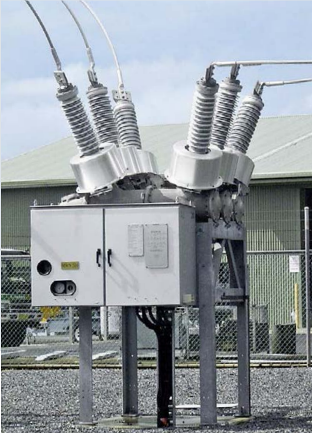
Fig. 11: SPS2/3AP1 DT 72.5 kV
