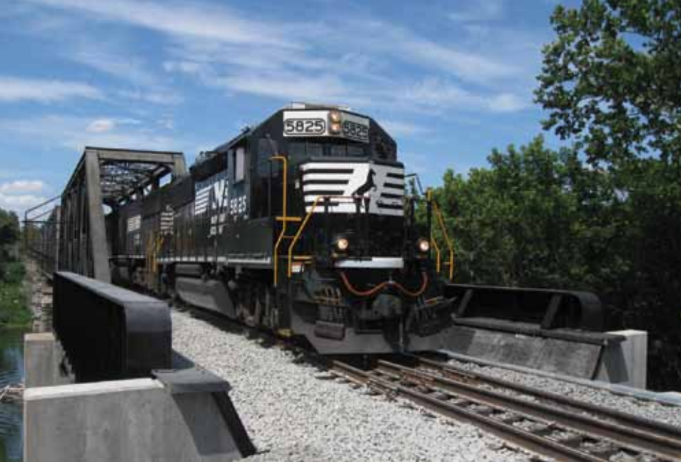
■ A train passes over the new bridge span at Riverton Junction. Michael Breen , NS project engineer design and construction, took the photograph, which appears in the 2011 NS calendar.
