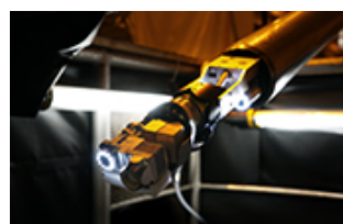
System for investigating inside the primary containment vessel of Unit 2
