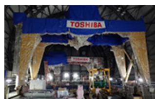
Fuel removal system of Unit 3 (Photo courtesy of TEPCO)
