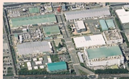
Himeji Operations-Semiconductor seeks to conserve energy in the clean room
