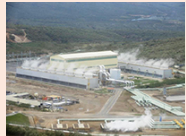
Olkaria IV Geothermal Power Plant in Kenya
