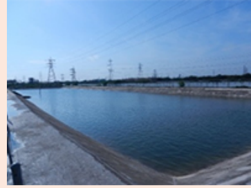
Reuse of rainwater and wastewater at Toshiba JSW Power Systems Pvt. Ltd. in India
