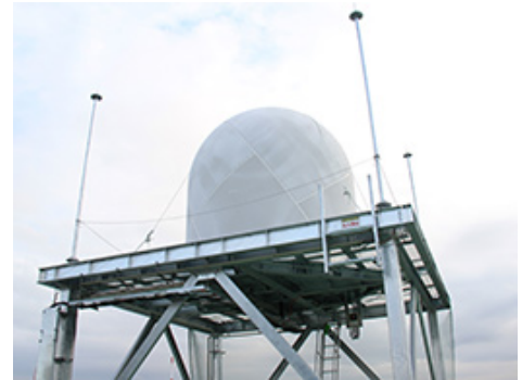
Multi-parameter phased array weather radar (MP-PAWR)
