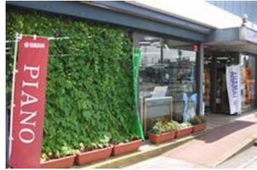
Green Eco Curtain at Yamaha Music Retailing Co., Ltd.'s Kurashiki store
