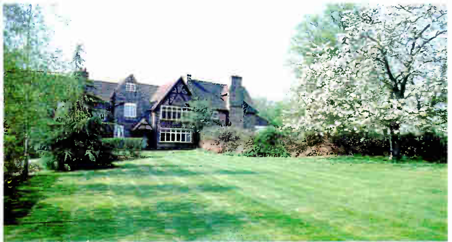
Farmyard Recording Studios, a residential facility 30 minutes from central London.
