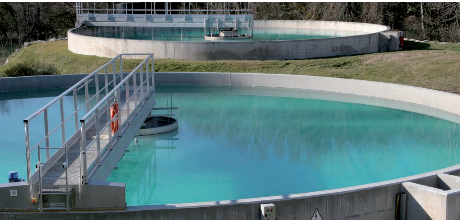
Water treatment plant, Rousset, France
