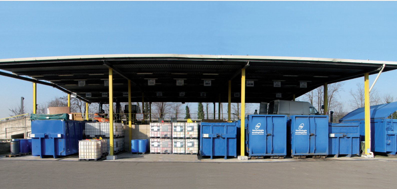
Waste sorting 'Eco Island', ST Agrate, Italy
