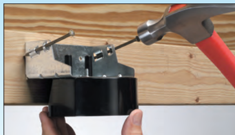
Nails to SINGLE JOIST
