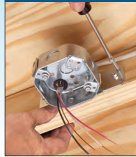
FBS415S/FBS420S Mount on SIDE of Joist
