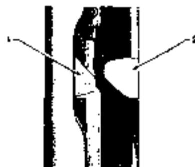
1—Female dovetail 2—Male dovetail
