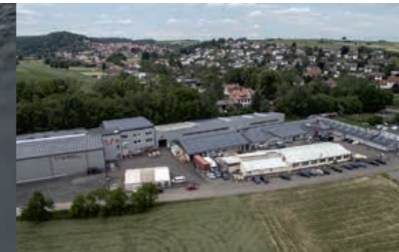
Headquarters, Rauschenberg, Germany
