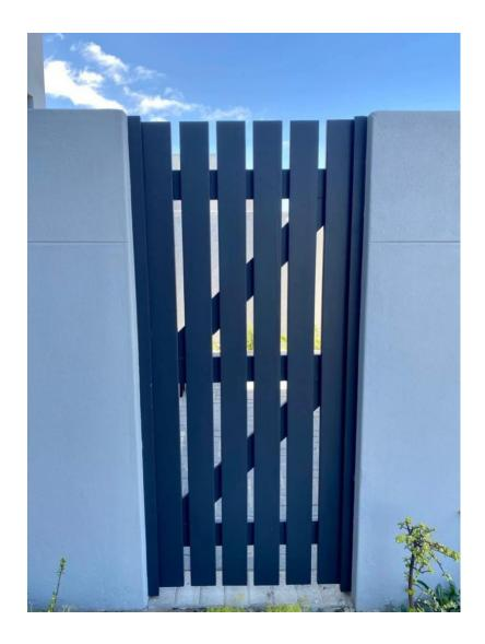
**Required dimensions/specifications:** Vertical timber planks should be the standard width of 105mm and the gaps between the planks should not be less than 25mm or more than 50mm.
