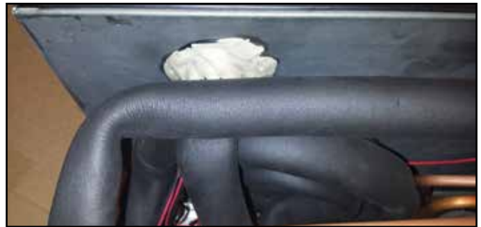
Figure 6-1.1. Sealing Compound (Inside)
