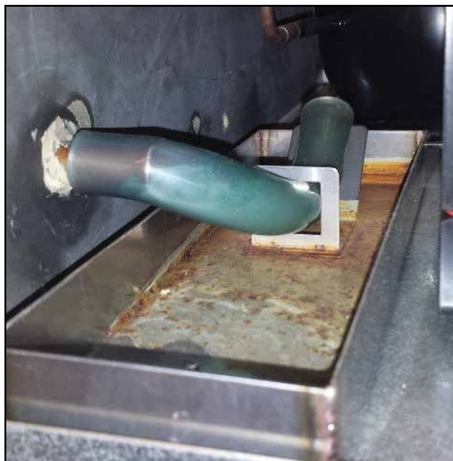
Figure 6-3. Evaporator Condensate Drain
