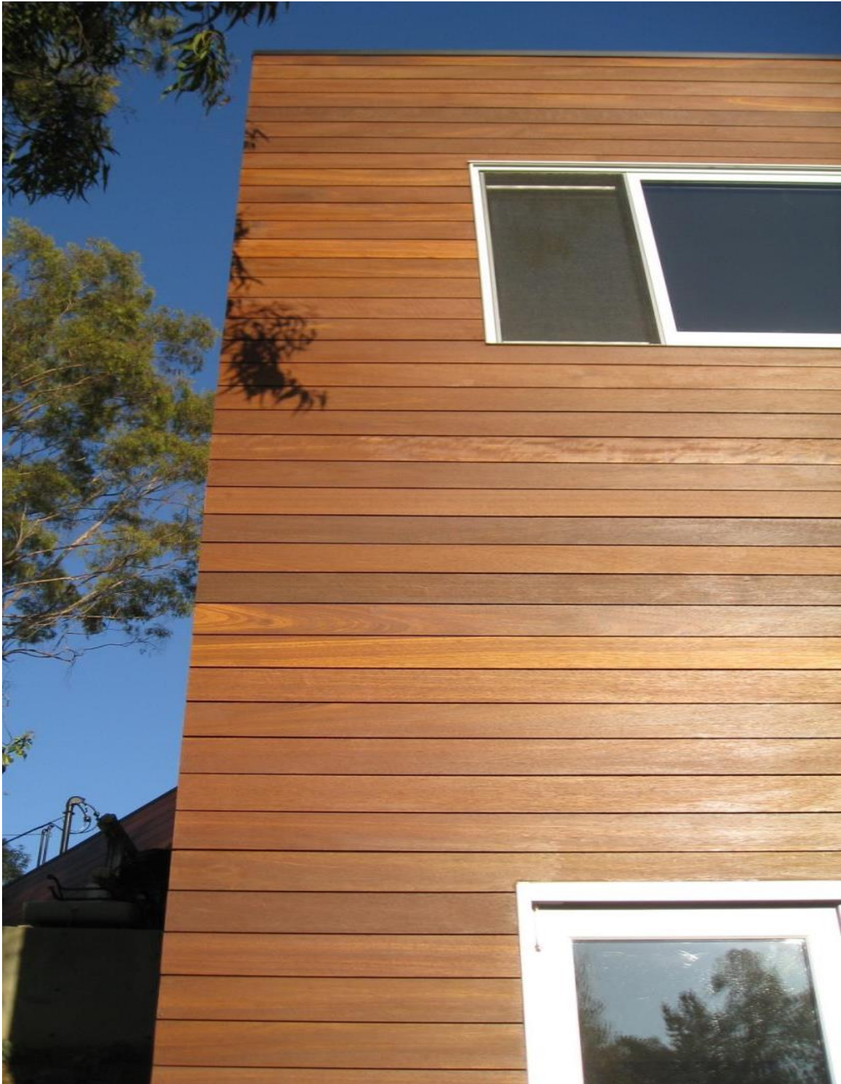
Residential rainscreen project in Southern California using 1x6 hardwood siding and mitered outside corners.
