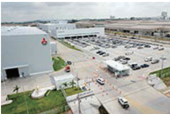
Mitsubishi Motors (Thailand) Co., Ltd. (MMTh)
