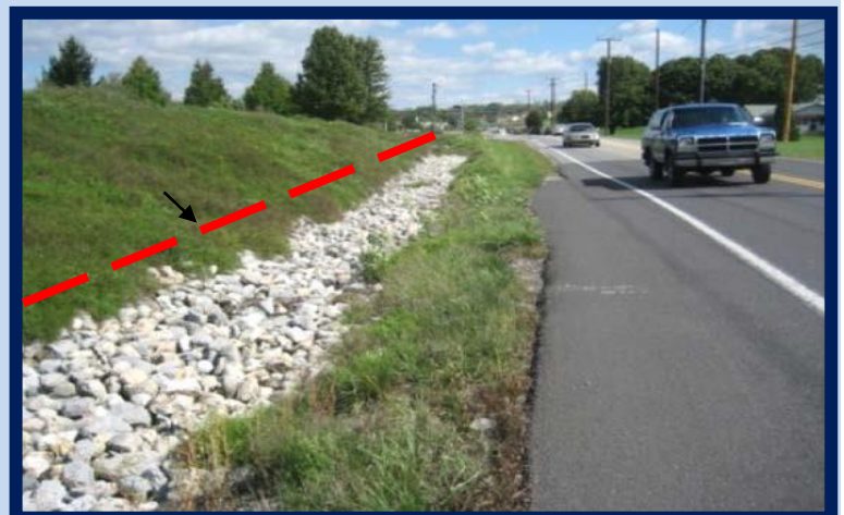
Figure 1.2.2- Storm water conveyed by parallel ditch along road.
