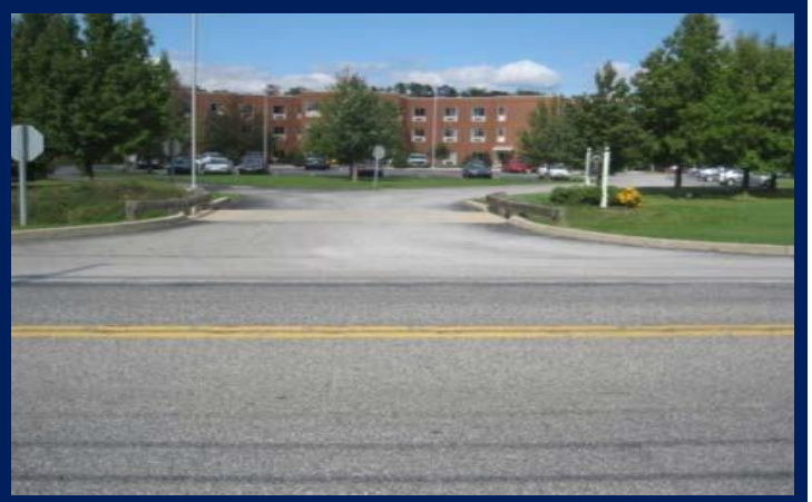
Figure 1.1.2- Culvert conveys water under driveway.
