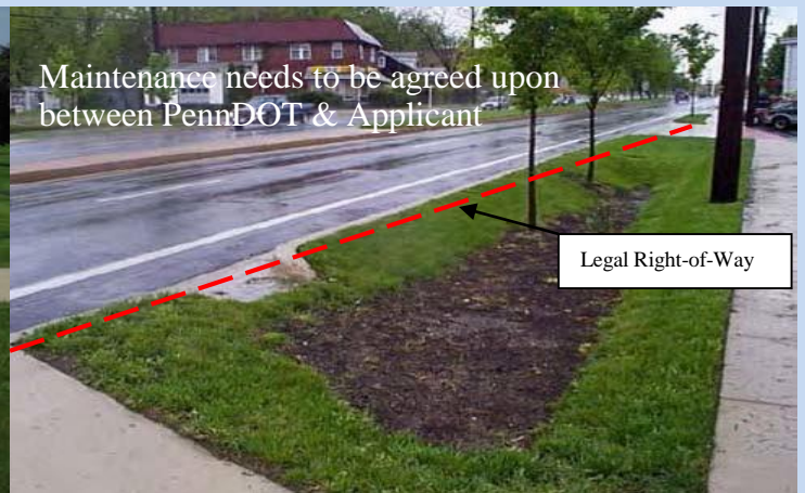
Figure 2.3.2- Alternative installation directs water to an infiltration trench off the right-of-way without the use of inlets and enclosed storm water facilities
