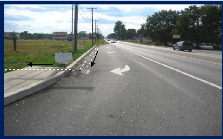
Figure 1.4.1- New enclosed surface storm water installed with curb gutter as part of widening for right turn lane.
