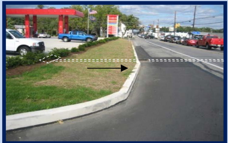
Figure 1.3.2- Site storm water directed into PennDOT Right-of-Way through enclosed surface storm water facilities tied into an existing inlet which is part of a larger storm water system.
