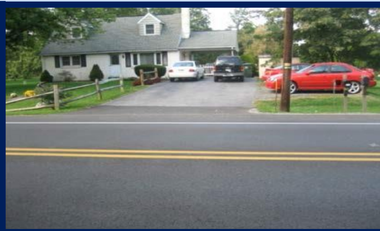
Figure 1.1.3- Storm water sheet flow across private driveway
