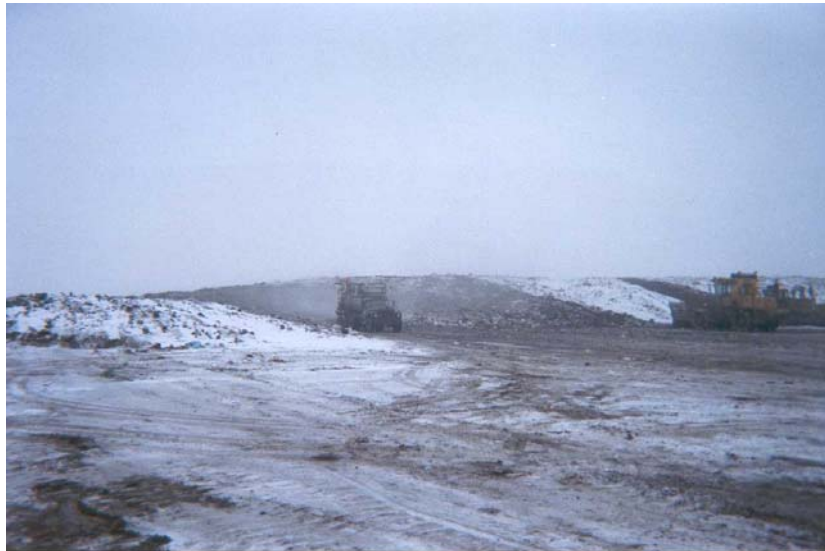
Photograph of Concover Being Applied to Working Face
