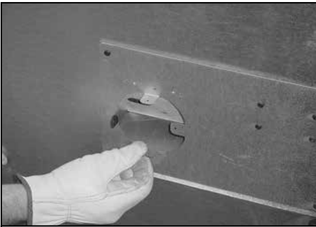
Figure 3.17 Bending Tabs on Outside Air Kit Collar
