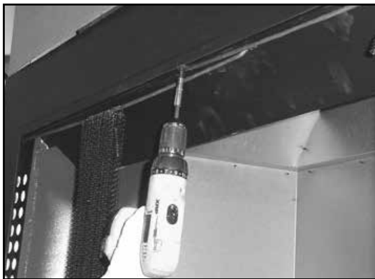
Figure 3.7 Remove Screen Rods
