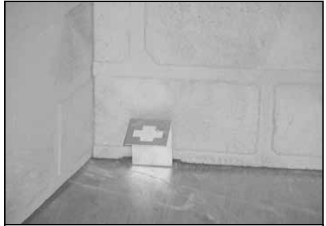
Figure 8.8 Grate Retaining Bracket in Place
