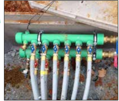
M-8400 GeoGreen™ mounted ground vault.
