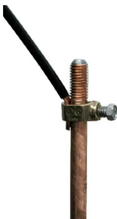
FIGURE 5-14. The #4 cable connected to the ground rod
