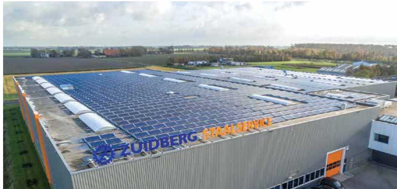
The Netherlands, 2MW
