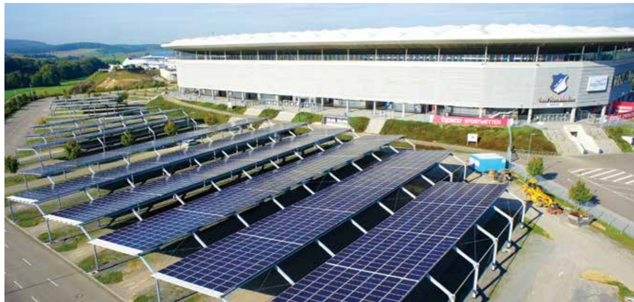
Germany, 1MW Carport of TSG Hoffenheim Stadium, Sinsheim
