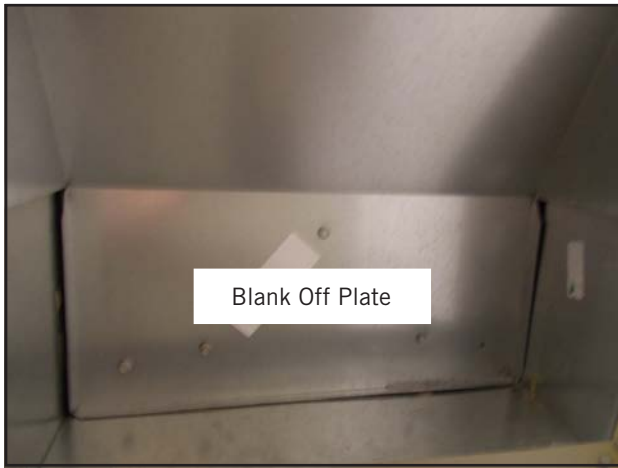
FIGURE 4 Remove Blank Off Plates (Both Sides)
