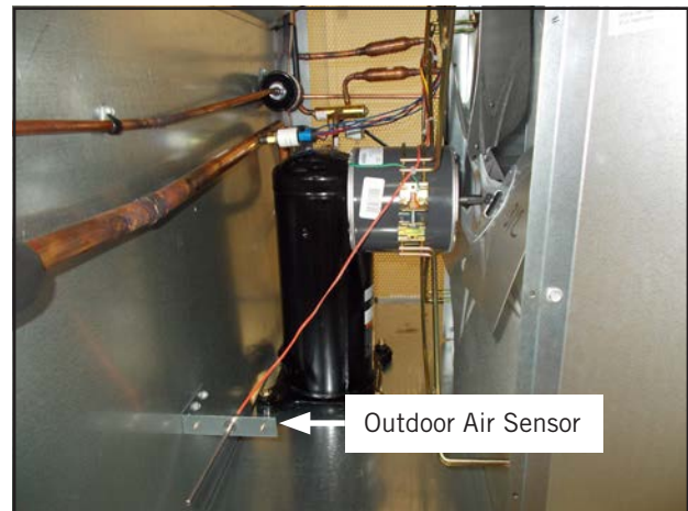
FIGURE 7 Install Outdoor Air Sensor
