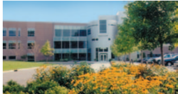
Parker Hannifin Corporation Headquarters Cleveland, Ohio
