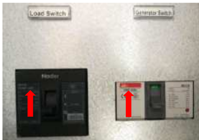
Figure 5.4 Load switch and diesel switch in switch-off status
