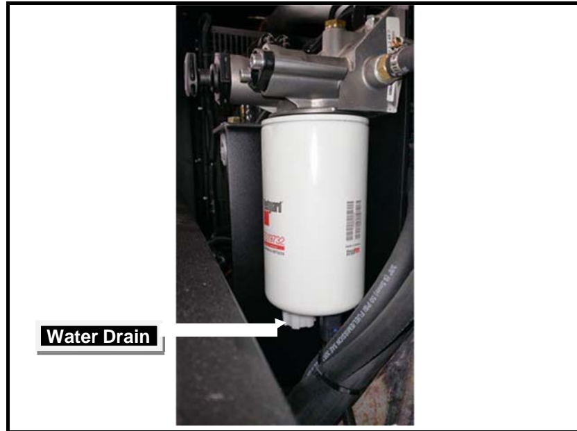
Figure 2-1-2 Fuel Lubricity Drain
