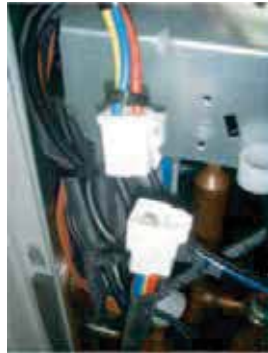
Figure 46: ARUN060GSS4 and ARUB060GSS4 Error No. 22 Compressor Terminal and Wiring Connections.
